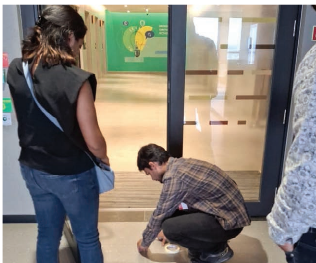
Figure 4 Site visits for checking progress
