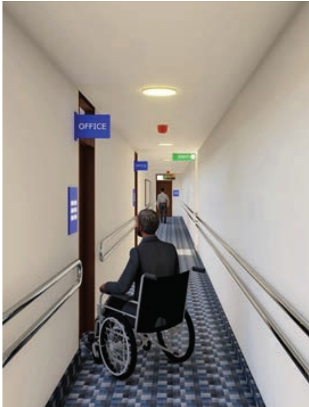
Figure 15 Internal corridors with adequate width and handrails
