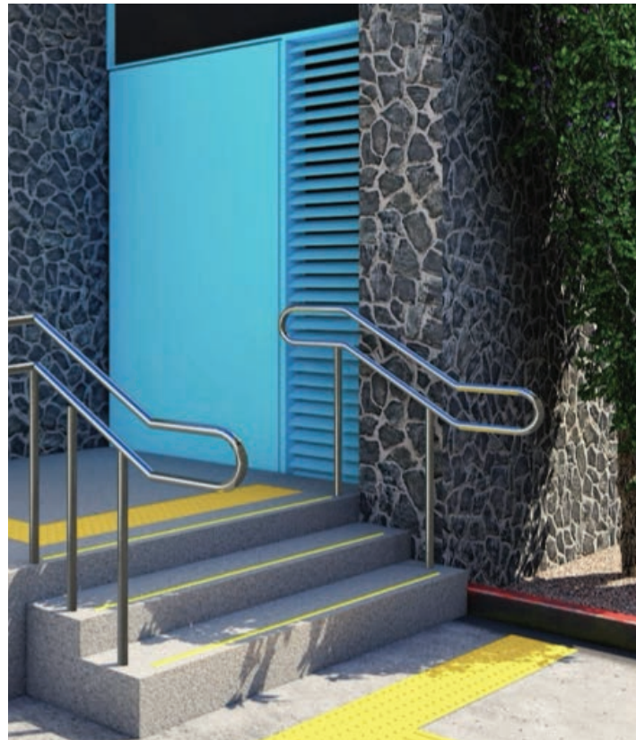
Figure 13 Steps with railings, colour contrasting nosing and tactile warning
